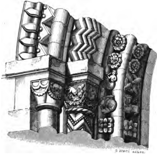
28. Part of South Doorway, Ifley Church, Oxon., c. 1160. Shewing rich Norman Ornament.
